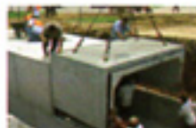
Split Box Culverts
