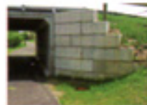
Bridge/Retaining Wall Blocks
