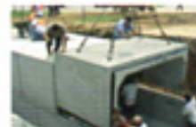
Split Box Culverts
